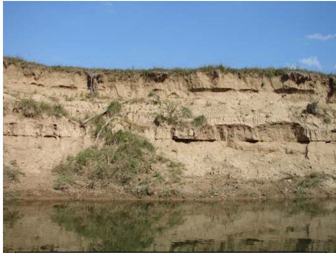
Streambank Erosion, Mainstem Saline River
