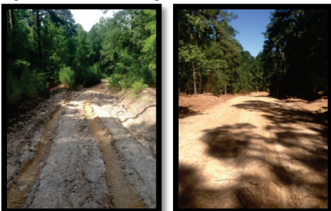
Figure 2: Phase II Scott Story Road Restoration. Before and After.
