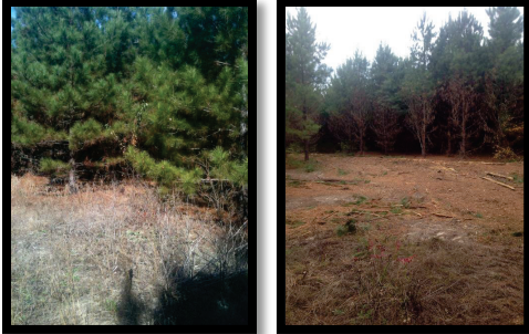
Figure 1: Phase II Mulching Work at Arkansas Oak. Before and After
